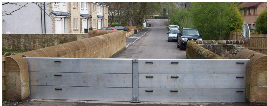
Figure 21. Batardeau multi-éléments - source 2leau-protection.com
